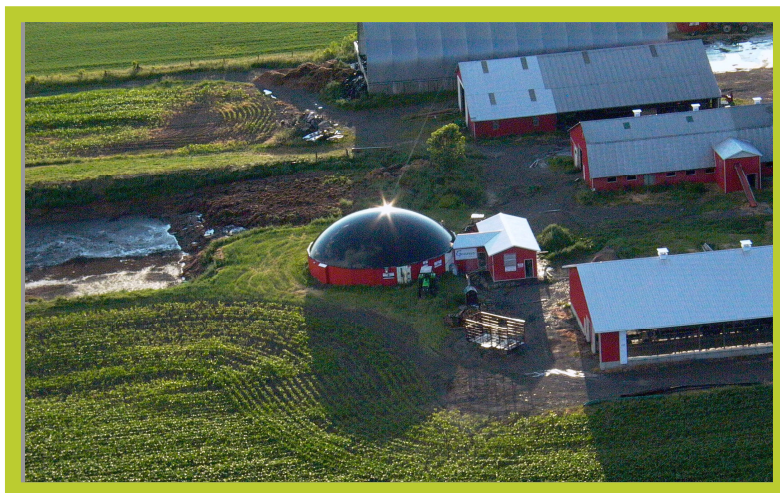
A CH-Four Biogas Inc. project in operation. St. Eugene, Ontario, Canada
